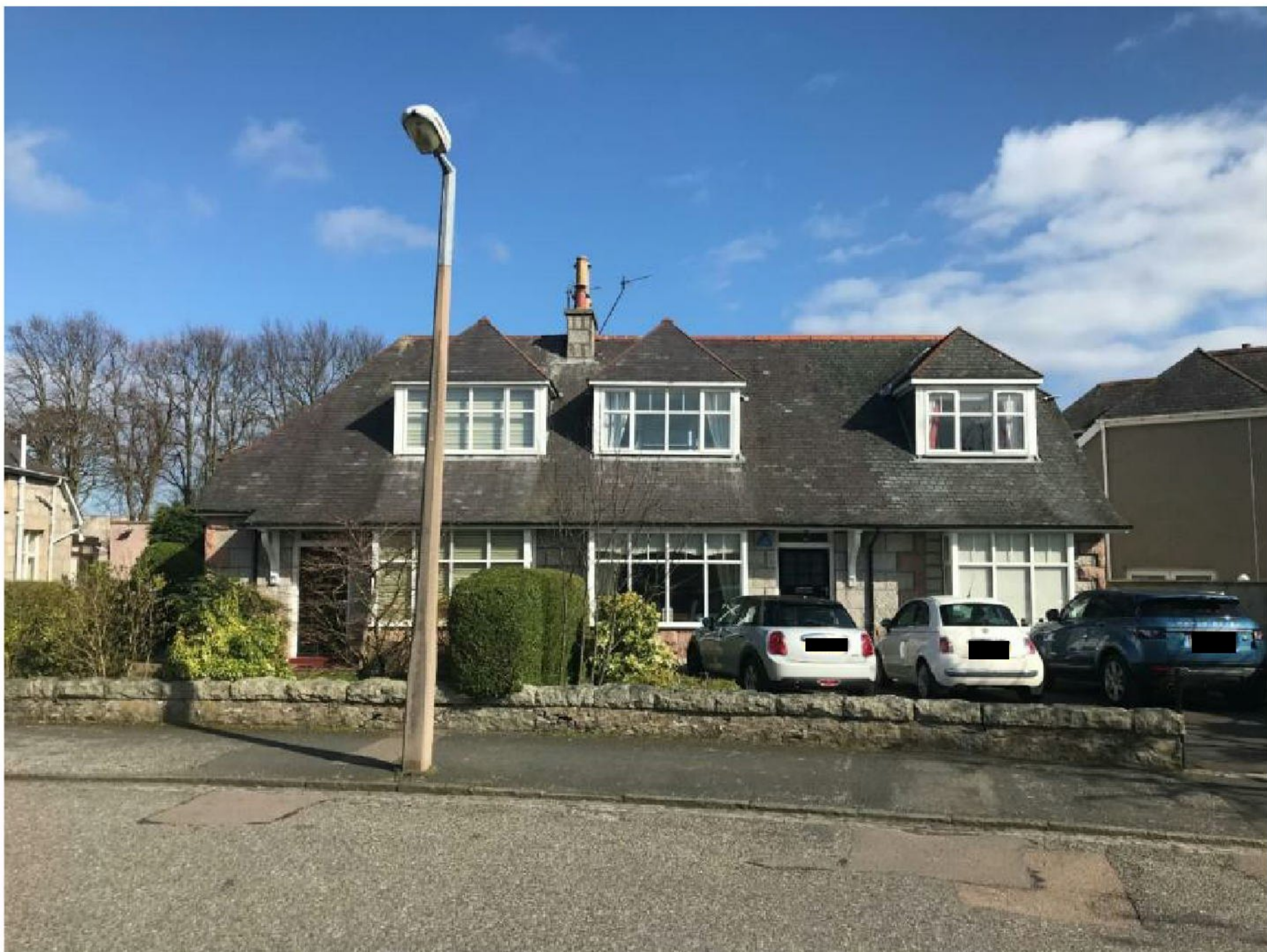
Image B: 13 & 15 Gordon Road (immediately adjacent to application property) – an identical roof profile to the proposal
