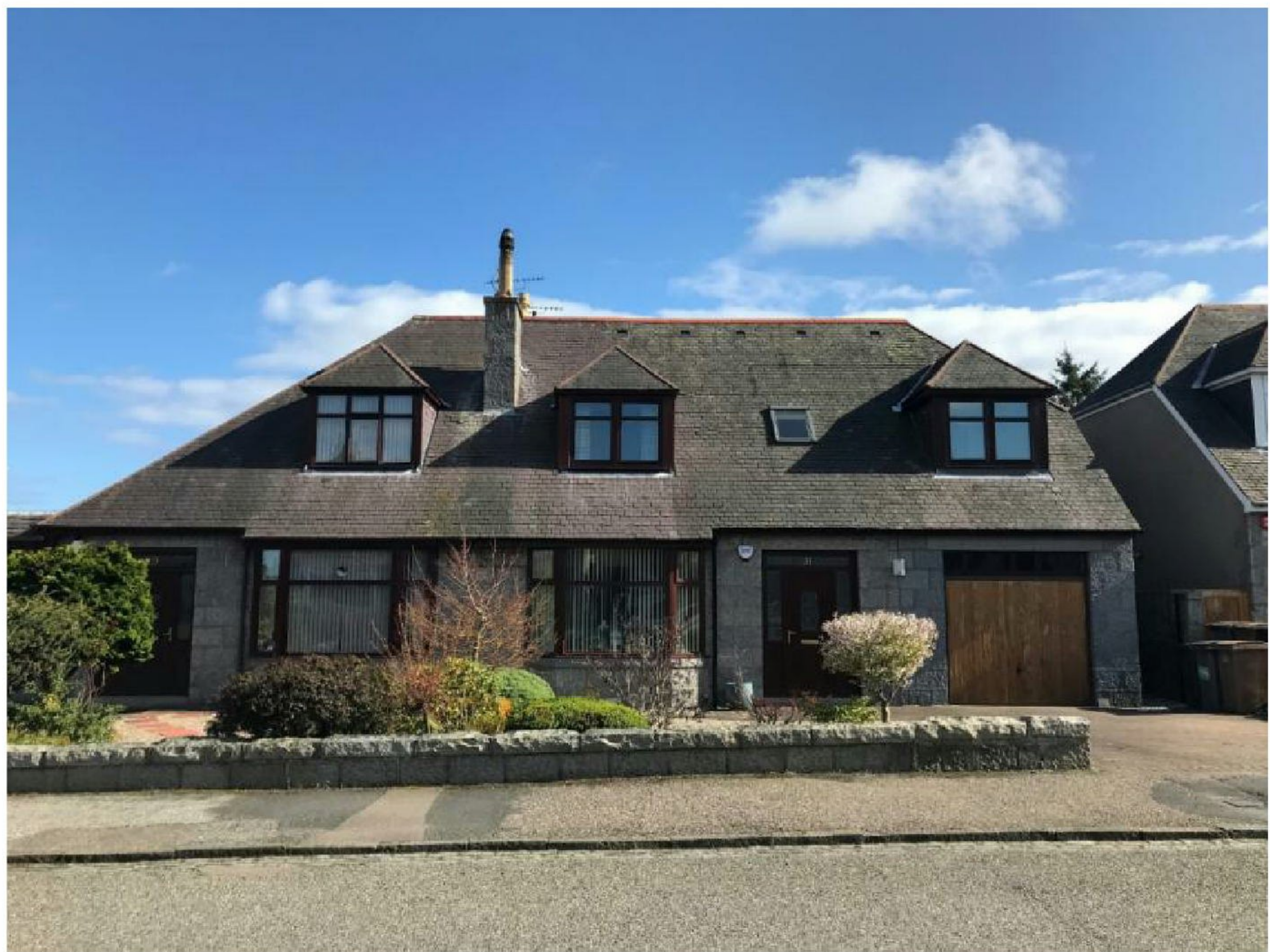
Image F: 29 & 31 Gordon Road – no. 31 has a 1/3 hip roof, again identical to the proposed roof profile at no. 11
