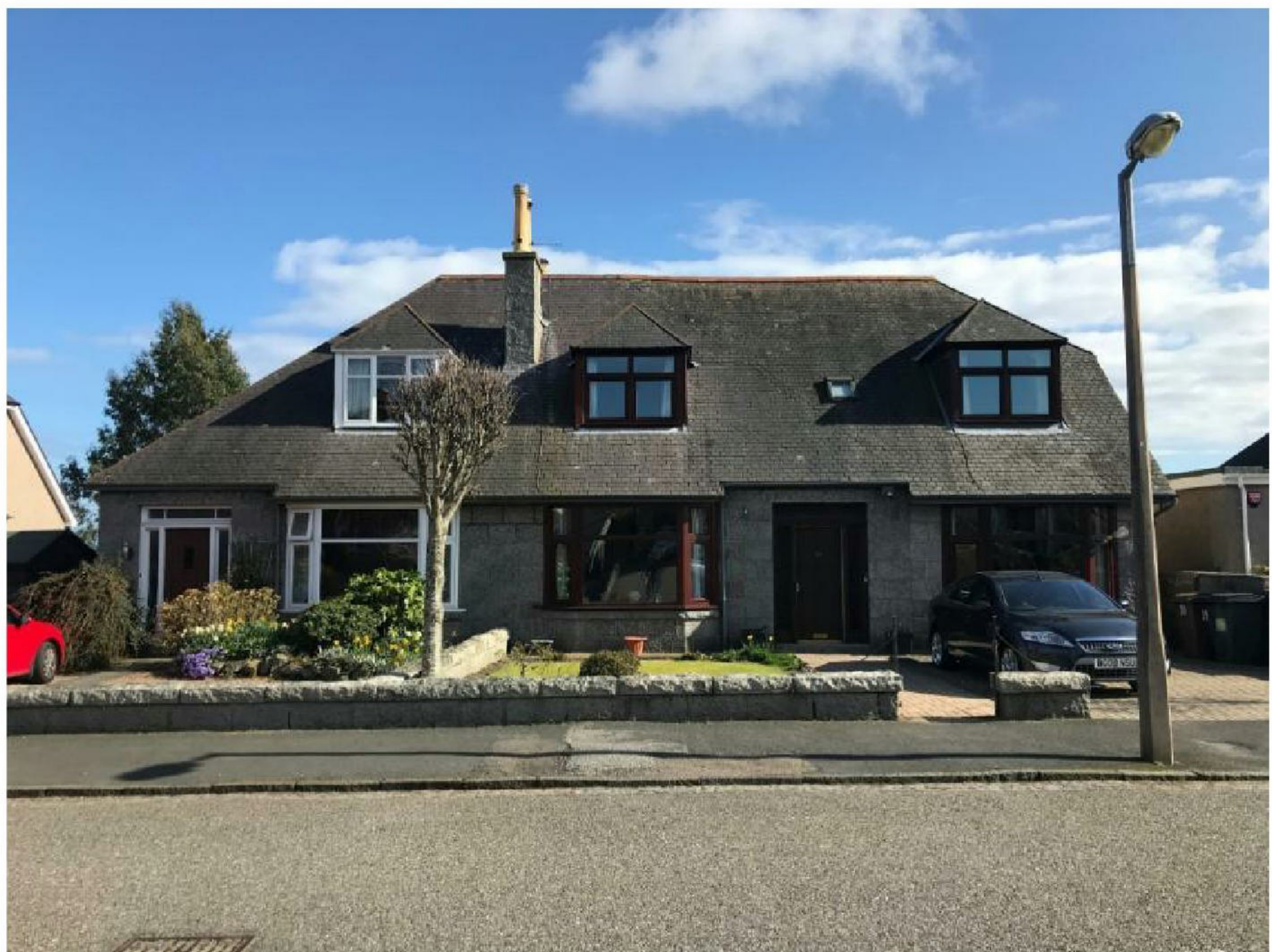
Image H: 37 & 39 Gordon Road – no. 39 has a 1/3 hip roof, again identical to the proposed roof profile at no. 11
