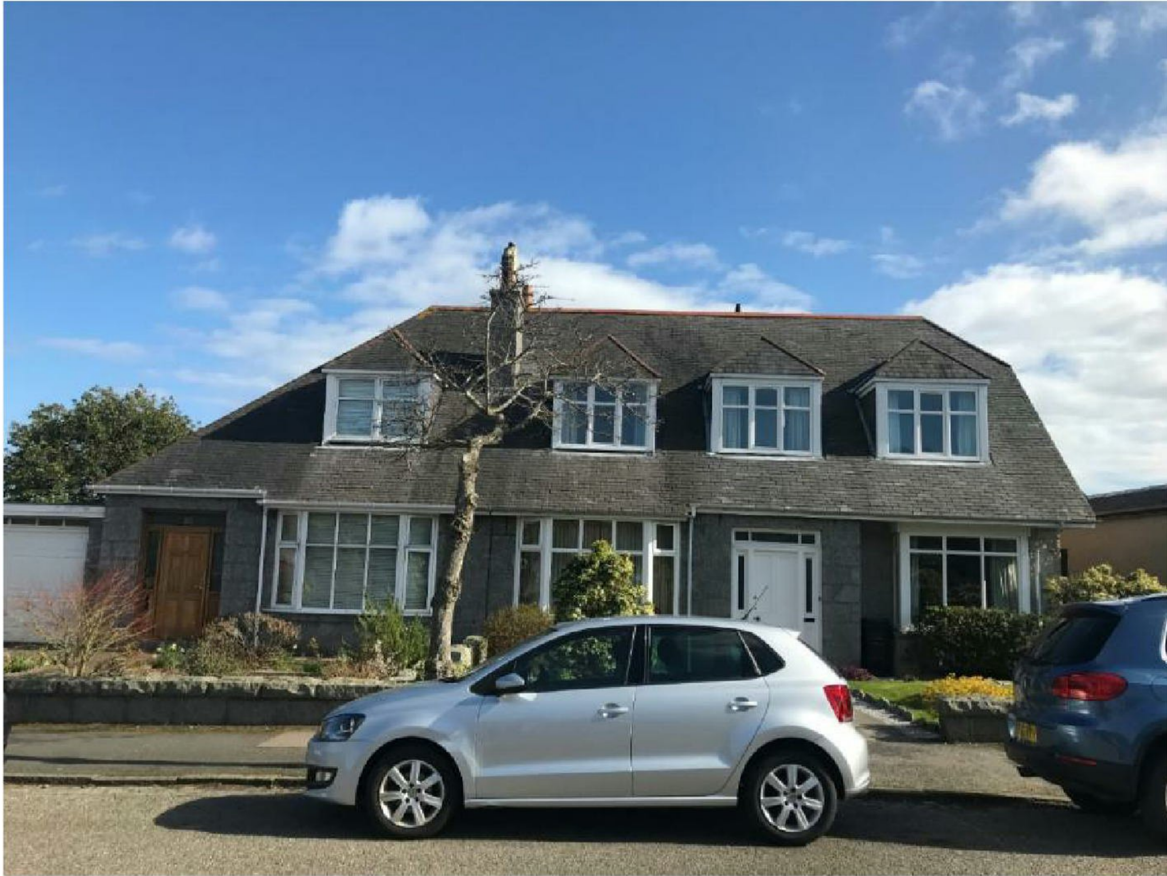
Image E: 25 & 27 Gordon Road – no. 27 has a 1/3 hip roof, again identical to the proposed roof profile at no. 11
