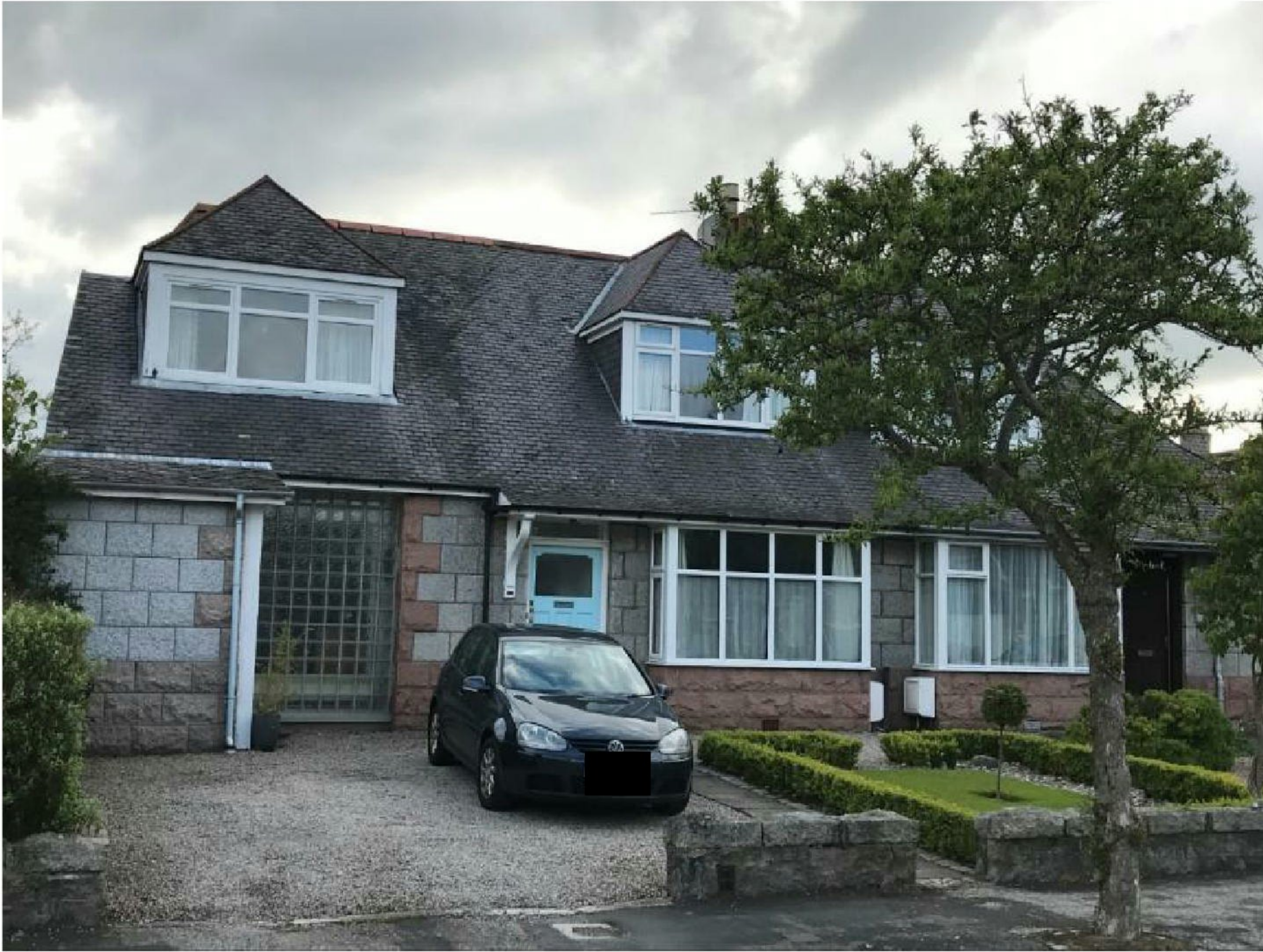
Image A: 2 & 4 Gordon Road (immediately opposite application property) – 1/3 hip roof profile to No. 4
