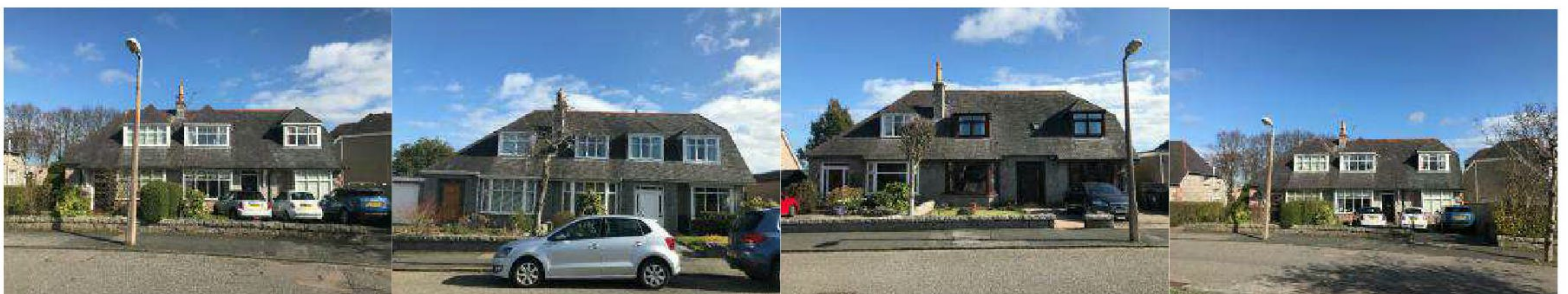
Further examples of half hip roofs to one side of semi-detached properties on Gordon Road
