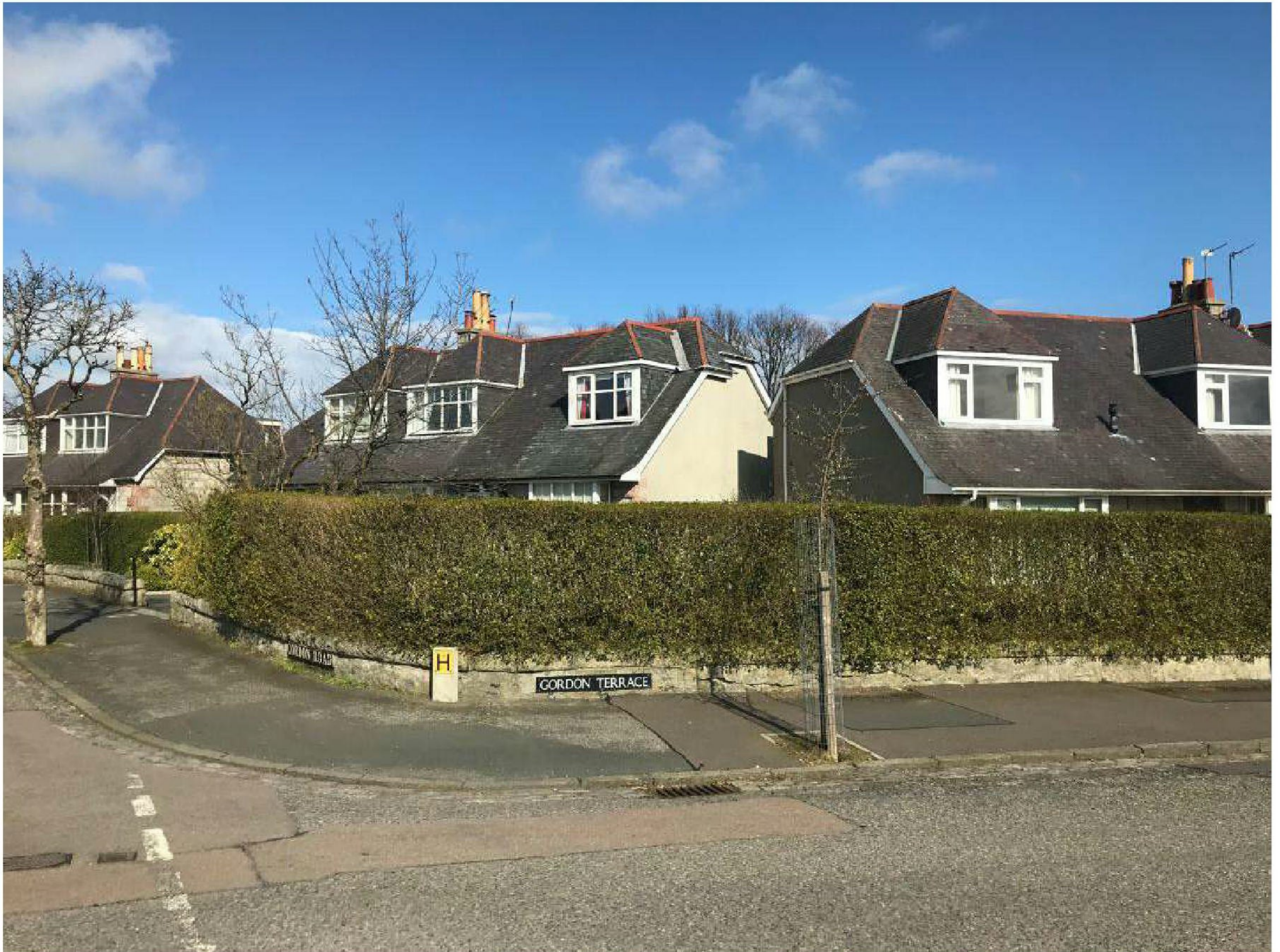
Photograph showing the application property on the left and two nearby extensions with half hip roofs
