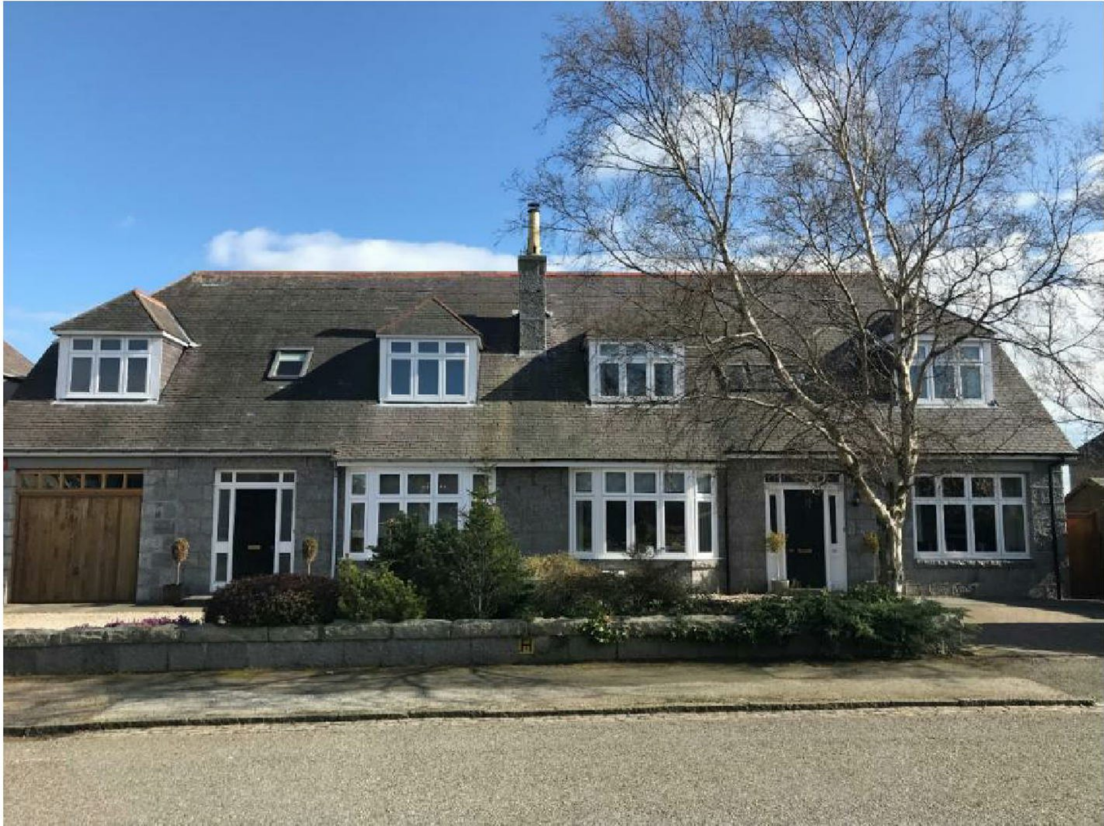
Image G: 33 & 35 Gordon Road – further examples of 1/3 hip roofs on the same side of the street
